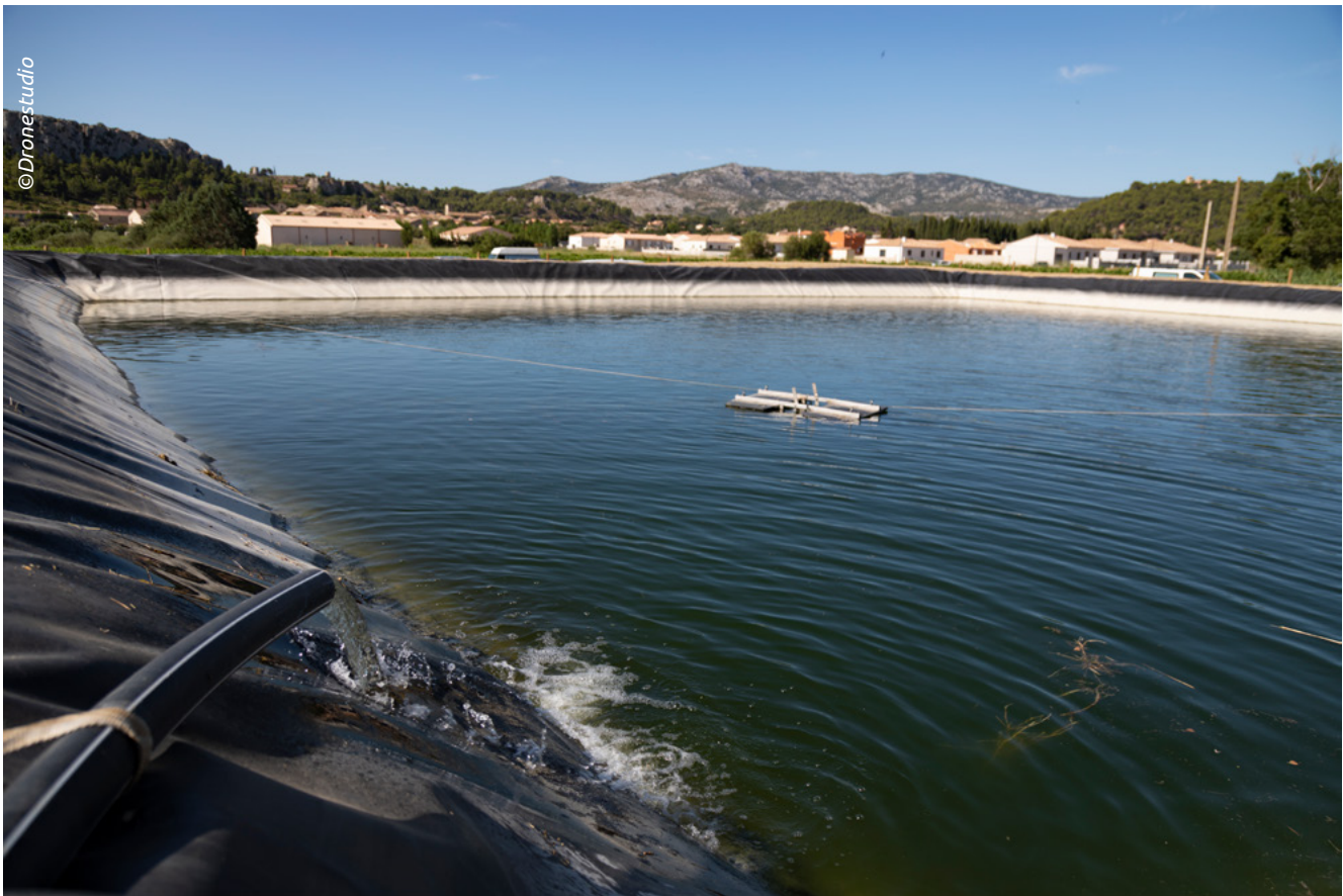
TWR facility in Roquefort-de-Corbières (Aude), operated by BRL Exploitation
